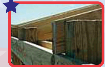
Double 2" x 8" (minimum) Top Plate. 2" x 10" or 2" x 12" used for spans 36' wide or over.
