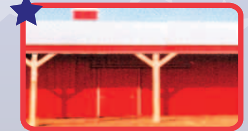
V-Braces are used on open walls, sheds, and porches.
